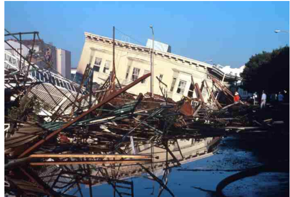
Collapsed and burned buildings in the Marina District, San Francisco. Loma Prieta, California, Earthquake October 17, 1989.
